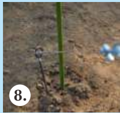
9. Connect iron rod with turnbuckle to fasten
