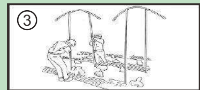
Penancapan pipa Arch
